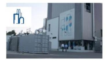
Sunfire's pilot plant in Germany has a capacity of 1 barrel per day (0.057 Million litres/year) and claims to save up to 3.14 tons of  $CO_2$  for each ton of fuel produced.
